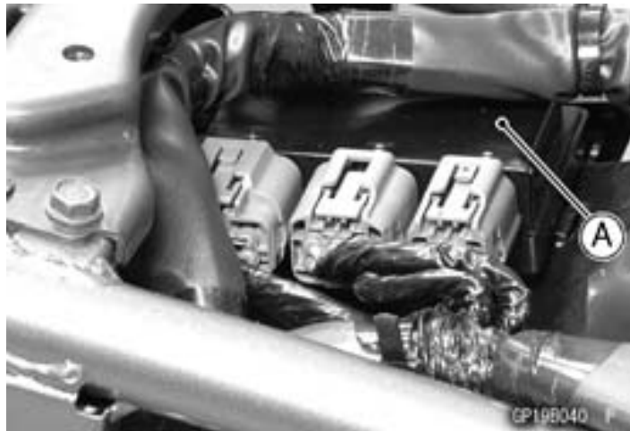
Relay Box – under fuel tank
